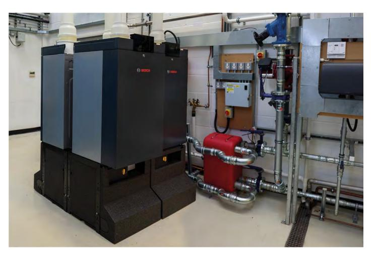
Available in outputs of 50, 65, 85, 100, 125 and 145kW. The Condens 7000 WP can be cascaded in banks of up to 6 boilers per bank providing up to 858.6kW at 50/30 per bank.
