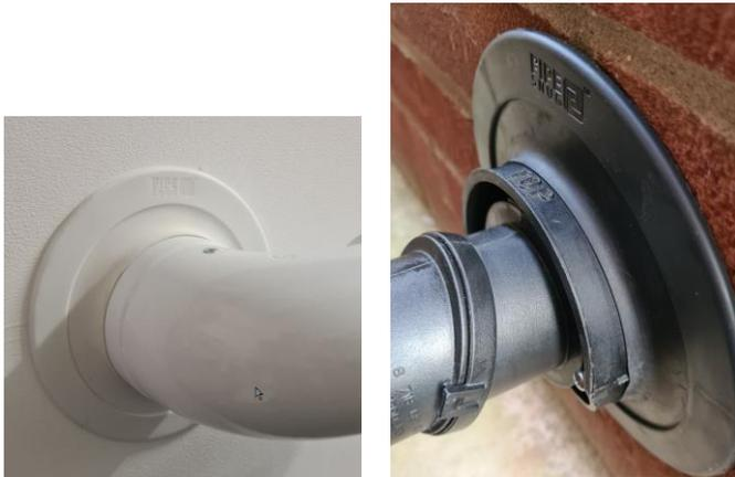
There are now products available which are specifically designed for sealing flues to the building fabric. They **can** remove the need for any further sealing or making good. We accept that these products can be used with our Oilfit & Condensfit II flues providing they are installed in place of, and in the situations described for our own wall sealing rings.
