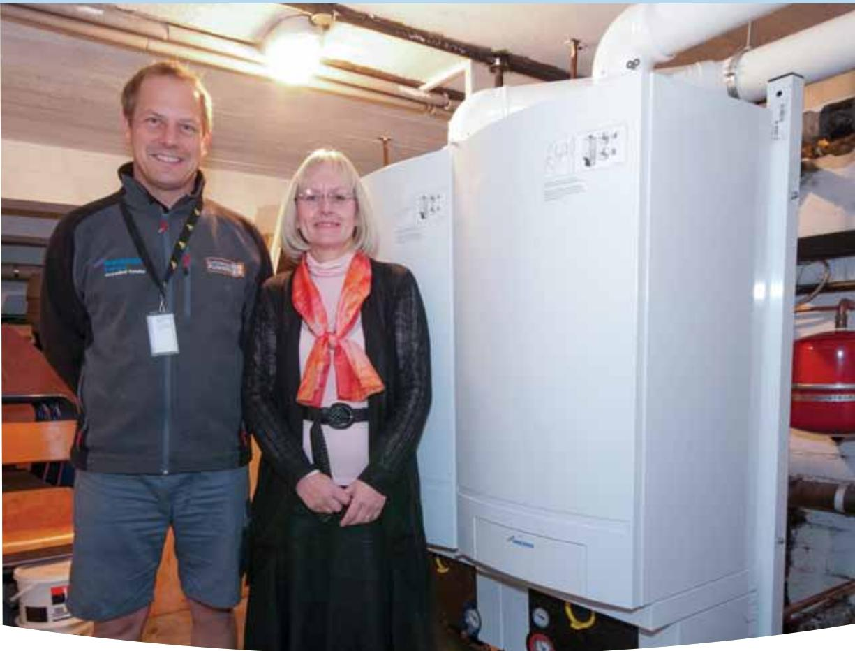
Another advantage of using a GB162 boiler is that it is incredibly quiet when in operation due to its low resistance and high quality insulation, making it ideal for inclusion in a church as it won't disturb the service.
