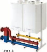
**Step 3:** Individual GB162 boilers are mounted securely on the framework.
